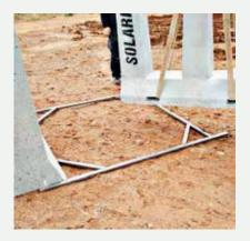
It is advisable to make the final positioning with the SOLARBLOC® H-S/18 structures being suspended by slings to obtain greater precision in the positioning step.
