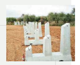
We can use a template or matrix with the necessary separation among each support. With this tool, the final placement of the structures SOLARBLOC® H-S/18 is made faster and more accurate.
