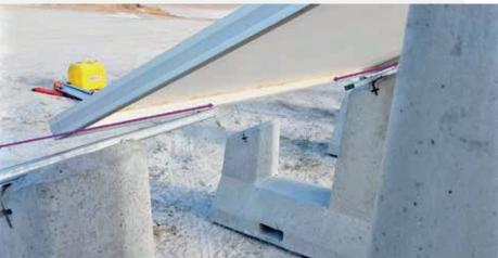
Mark the placement of each SOLARBLOC® H-S/18 and measure the height differences that will be present at each structure baseline. This is needed to determine the actions that will be carried out before the final positioning of the structures depending on the tolerance. These actions will take place over the surface o later over the attachment fittings.
