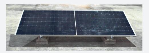
**Install all the rail extenders face up and use M8 × 50 mm bolts** to attach them to the SOLARBLOC structures. **Use end-clamps** to secure the panel in place (see the detail drawing below).
